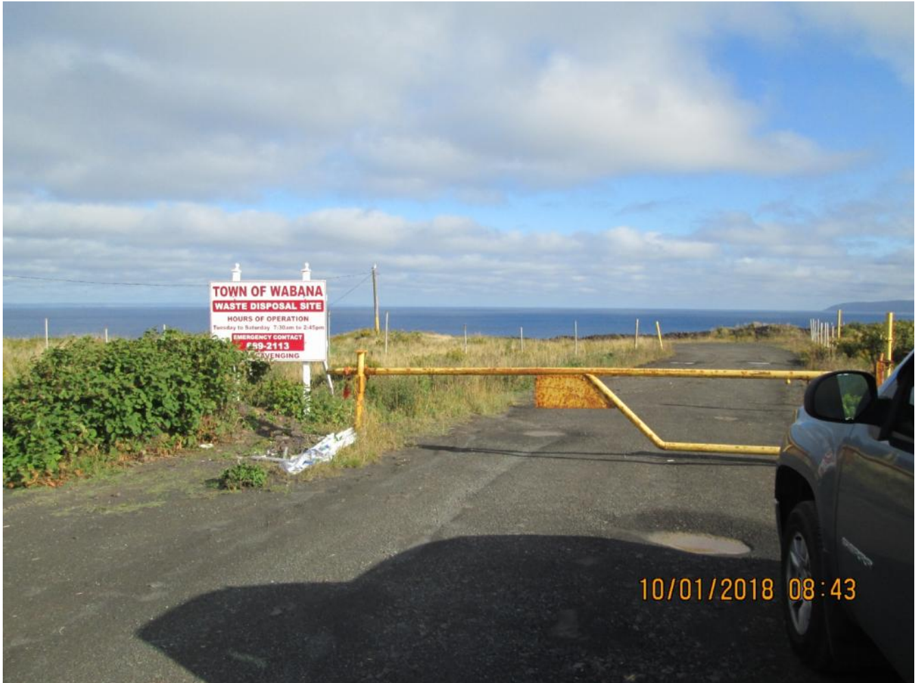
Photo 1 – Site #1 - Existing Bell Island Waste Disposal Site Entrance
