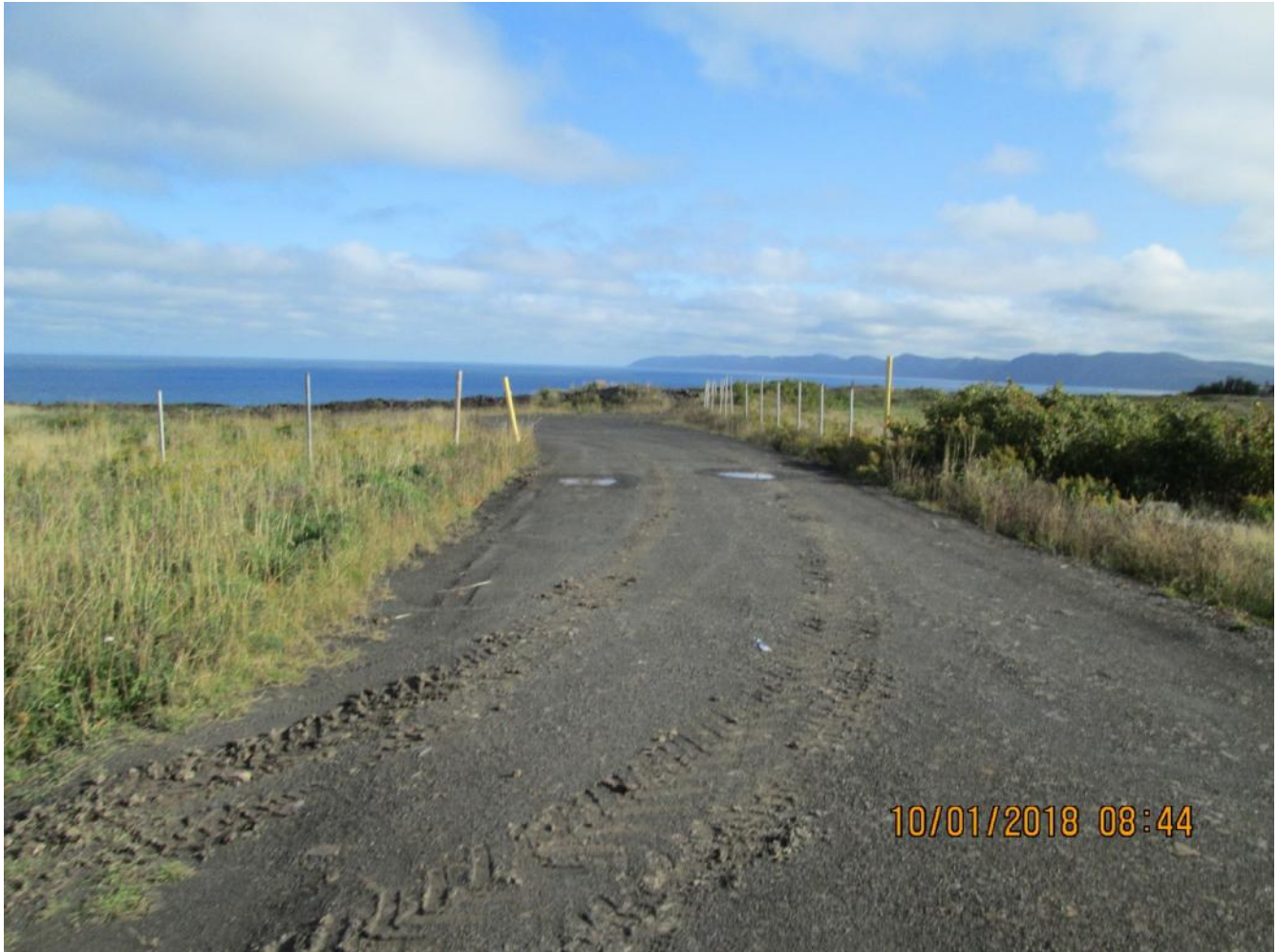
Photo 2 – Site #1 - Existing Bell Island Waste Disposal Site Access Road
