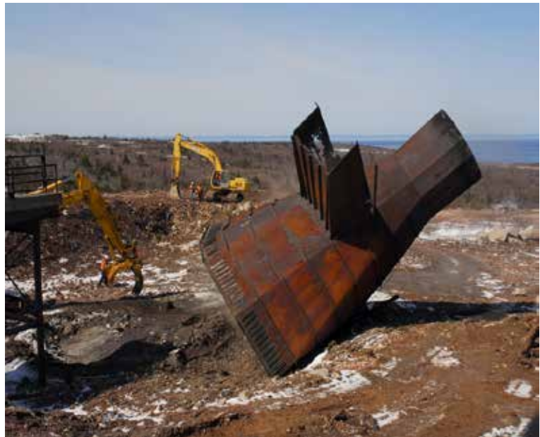
Incinerator in Old Perlican being dismantled and replaced with a waste recovery facility
